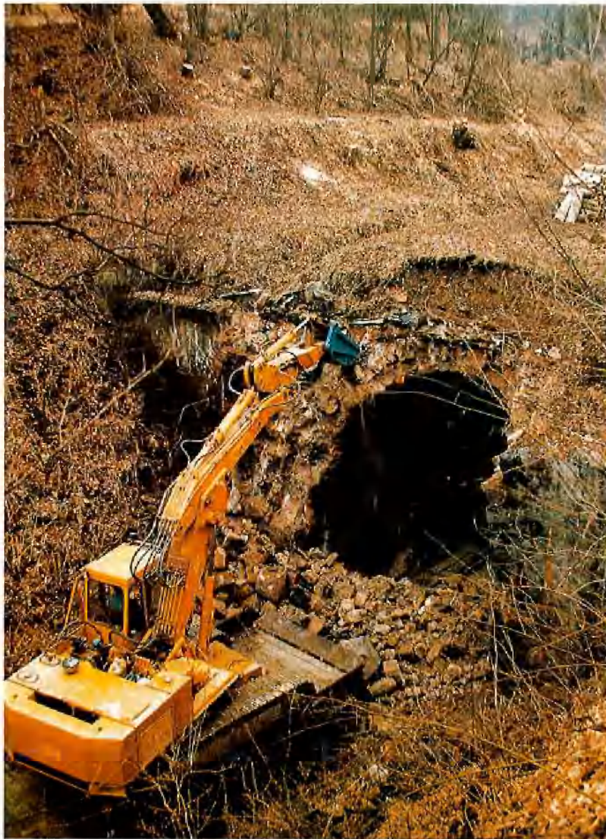
Portalabbruch Waldmichelbacher Tunnel
