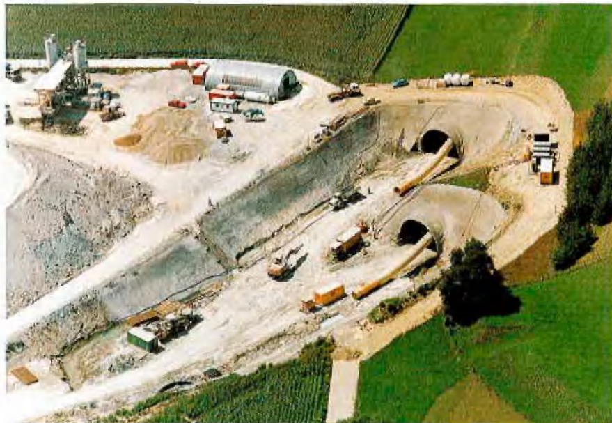
Westportal Terndorfer Tunnel
