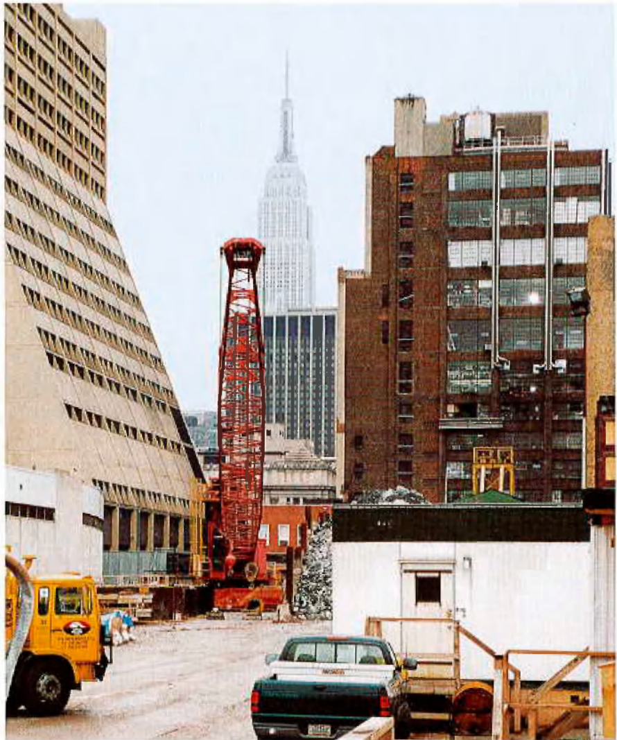
Baustelle in Manhattan
