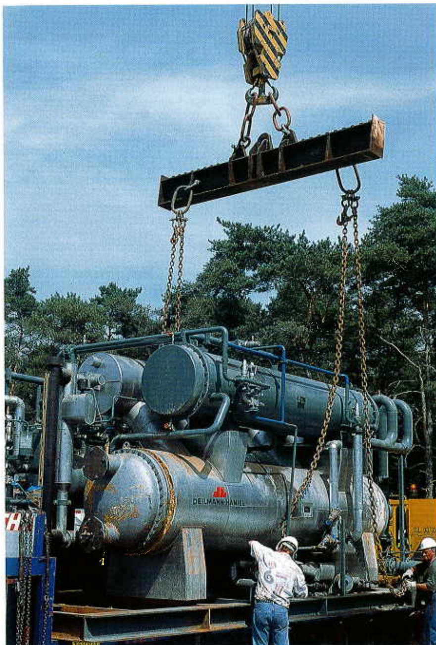
Montage der Gefrieraggregate
